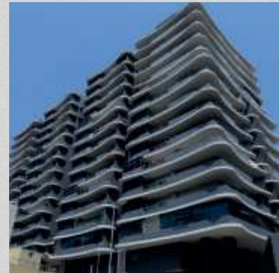
VIP TOWERS (COMPLETED) SIRIPURAM
